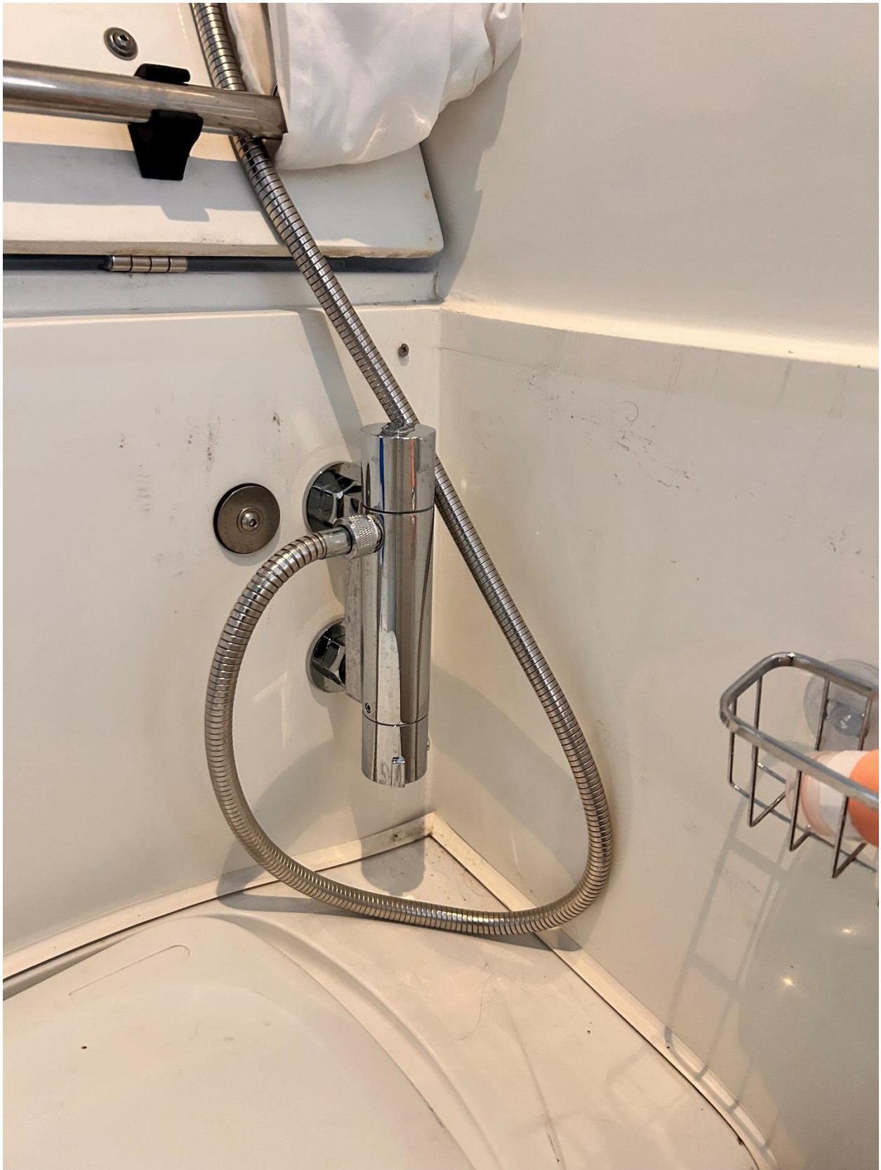
Figure 15: Thermostatic Shower Valve
